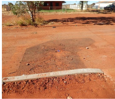
Photo 4 - Reconstruction of failed pavement
