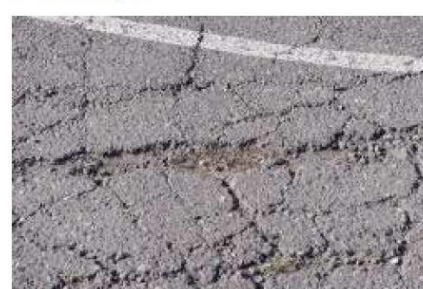
Localised cracking
