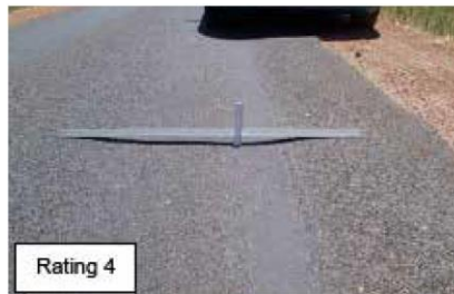
Heavy rutting (average depth 20 - 30 mm.)
