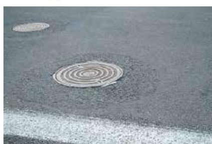
Poor patch repair
