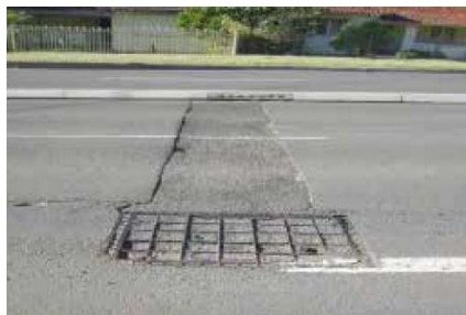
Poor trench repair
