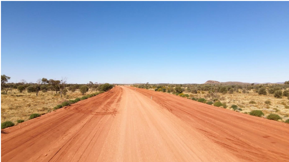
Caption: Works in progress on stages 1 and 2.
