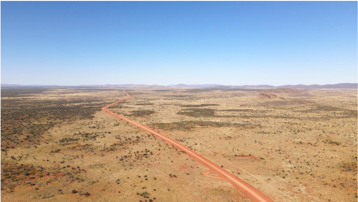
Caption: Overview of the site of the completed works.
