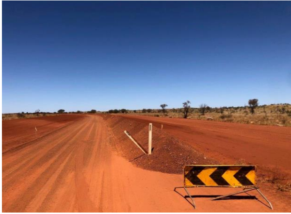
Caption: Wanarn Road, works in progress
