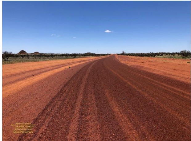
Caption: Wanarn Road, works complete.
