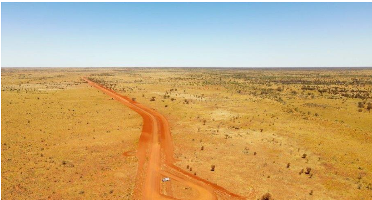
Caption: Wanarn Road, aerial view of completed works
