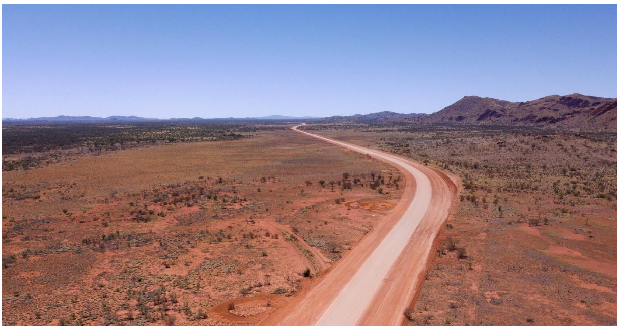
Caption: Papulankutja Road, aerial view of completed works
