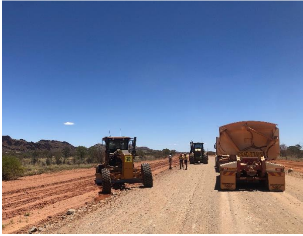
Caption: Papulankutja Road, works in progress
