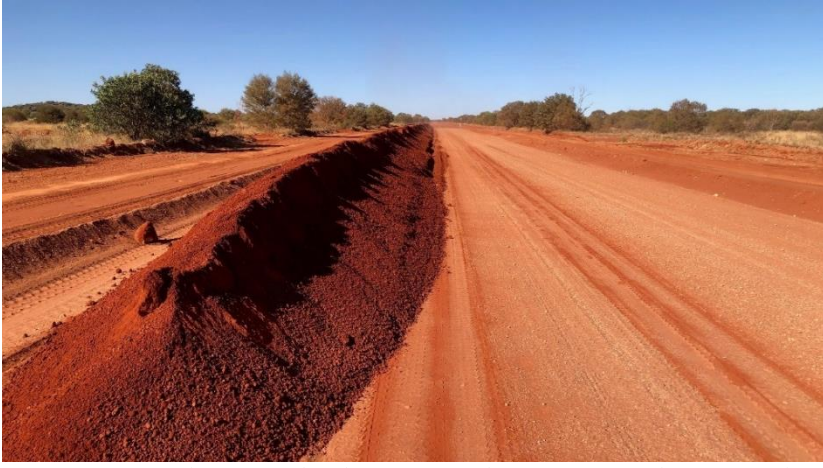
Caption: Completion of the drainage and formation widening works.
