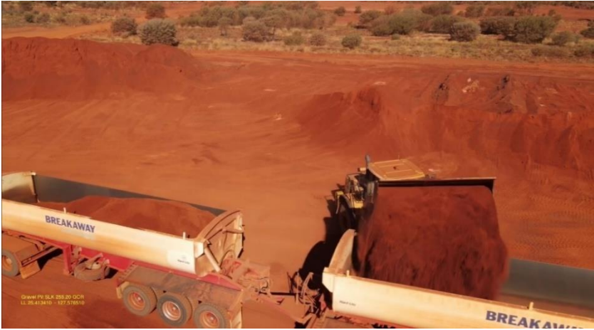
Caption: Supply of gravel for the road overlay
