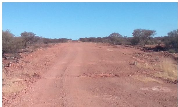
Caption: Tjirrkarli Road prior to start of works
