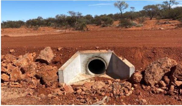
Caption: Tjirrkarli Road after installation of the culverts
