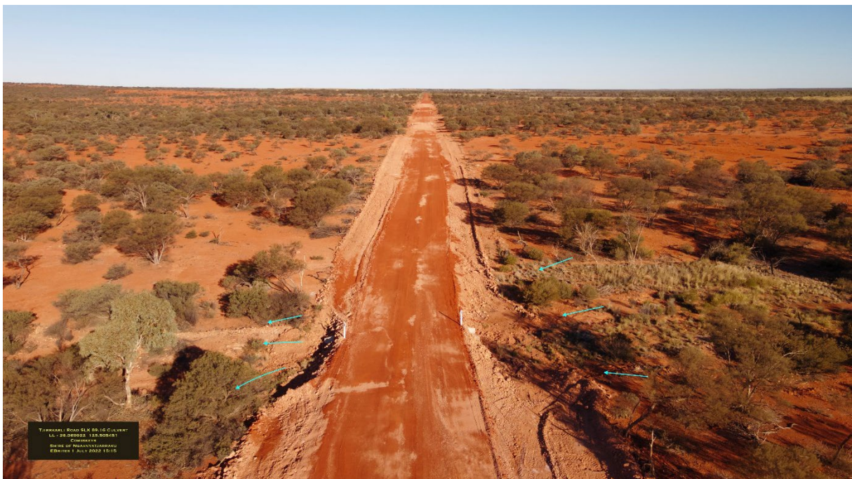
Caption: Tjirrkarli Road, aerial view of completed works
