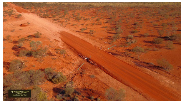
Caption: Tjirrkali Road, works complete.
